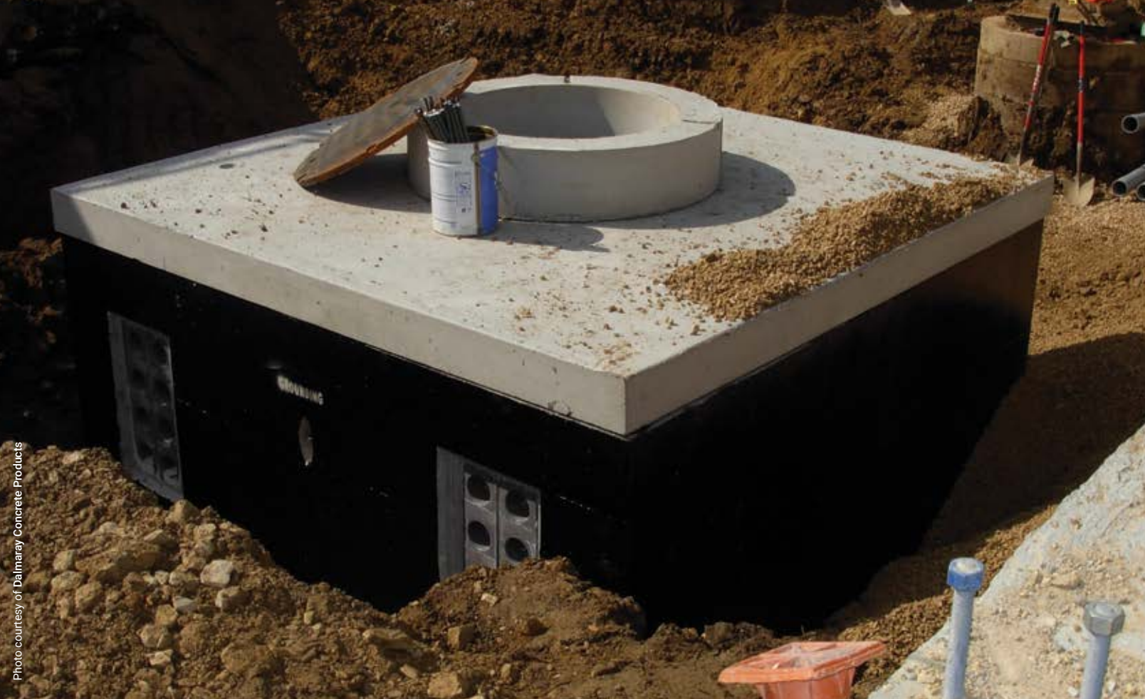
By using steel fibers in their mix, Dalmaray Concrete Products was able to reduce production time on precast electrical vaults for a Google Data Center project.
