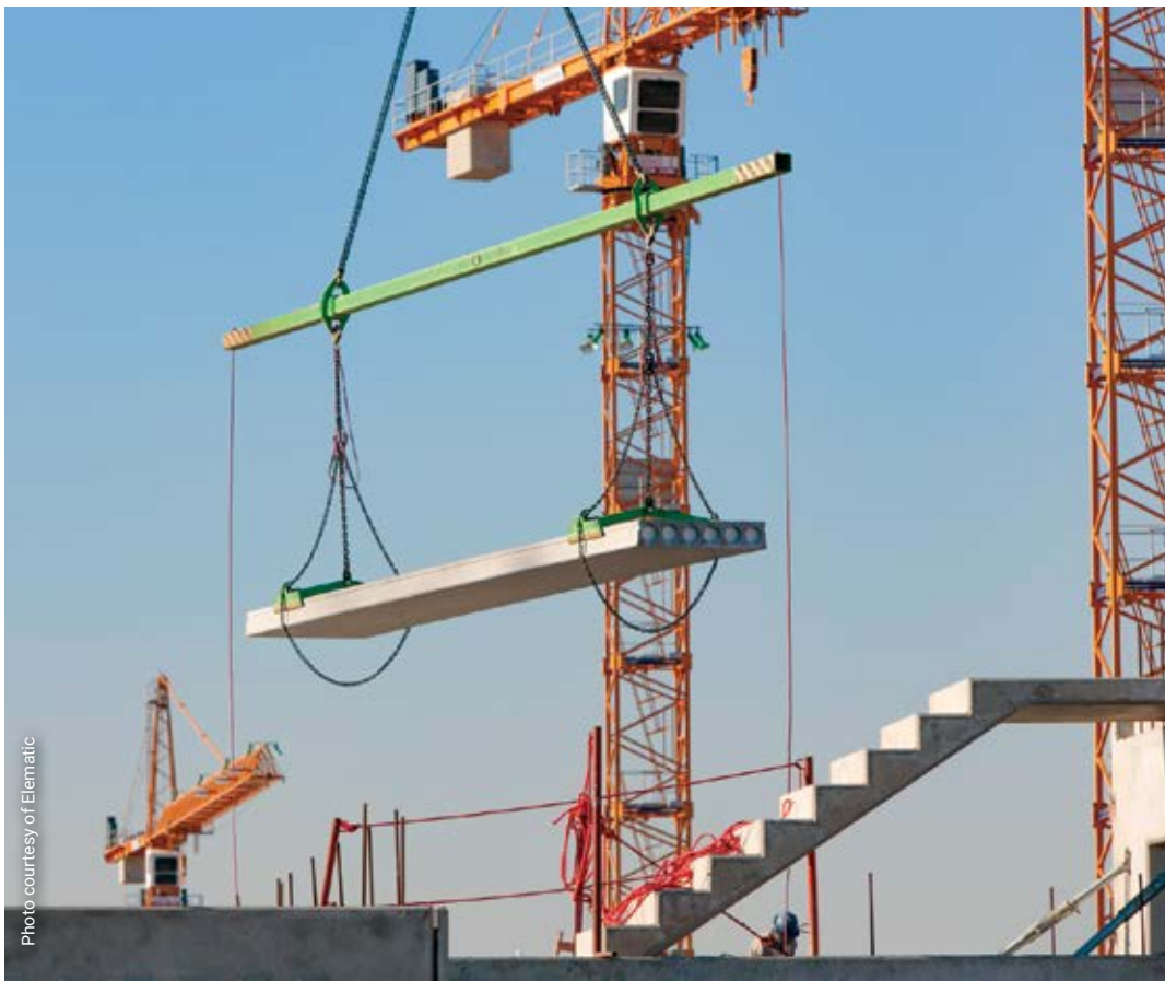
More than 1,000 hollowcore slabs are installed in each tower.
