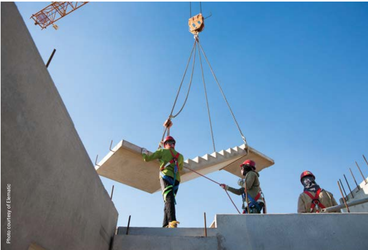
Each of the towers is constructed with 58 precast concrete staircases.
