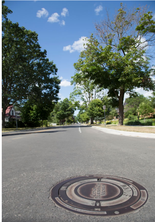
Traverse City has installed SELFLEVELs as part of their effort to keep streets smooth
