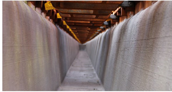
With the forms removed, the trench is complete.
