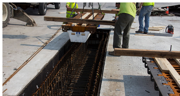
10-ft assembly is set into trench prepared with rebar cages.
