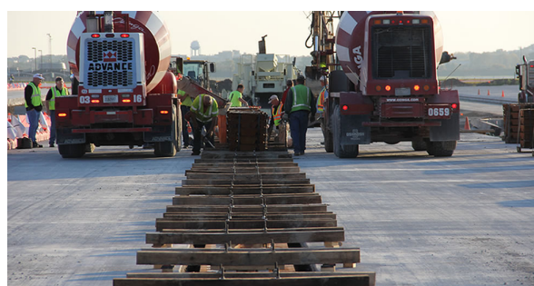
With the 4x4s holding the assemblies on grade, the concrete is poured, 350-ft. in one morning.
