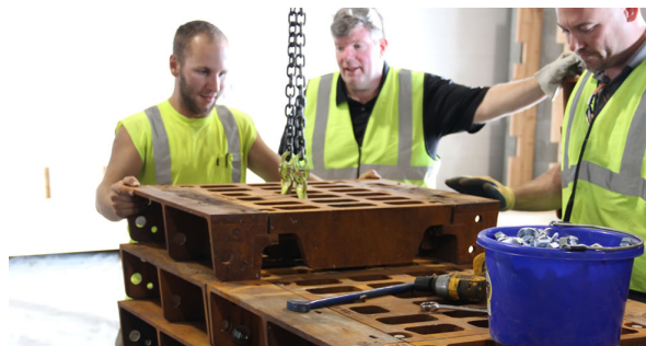
Experts from EJ on hand for installation support.
