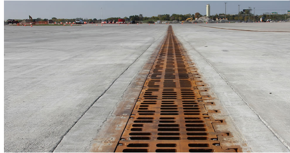
Trench aligns with the pavement grade, matching the slope precisely.
