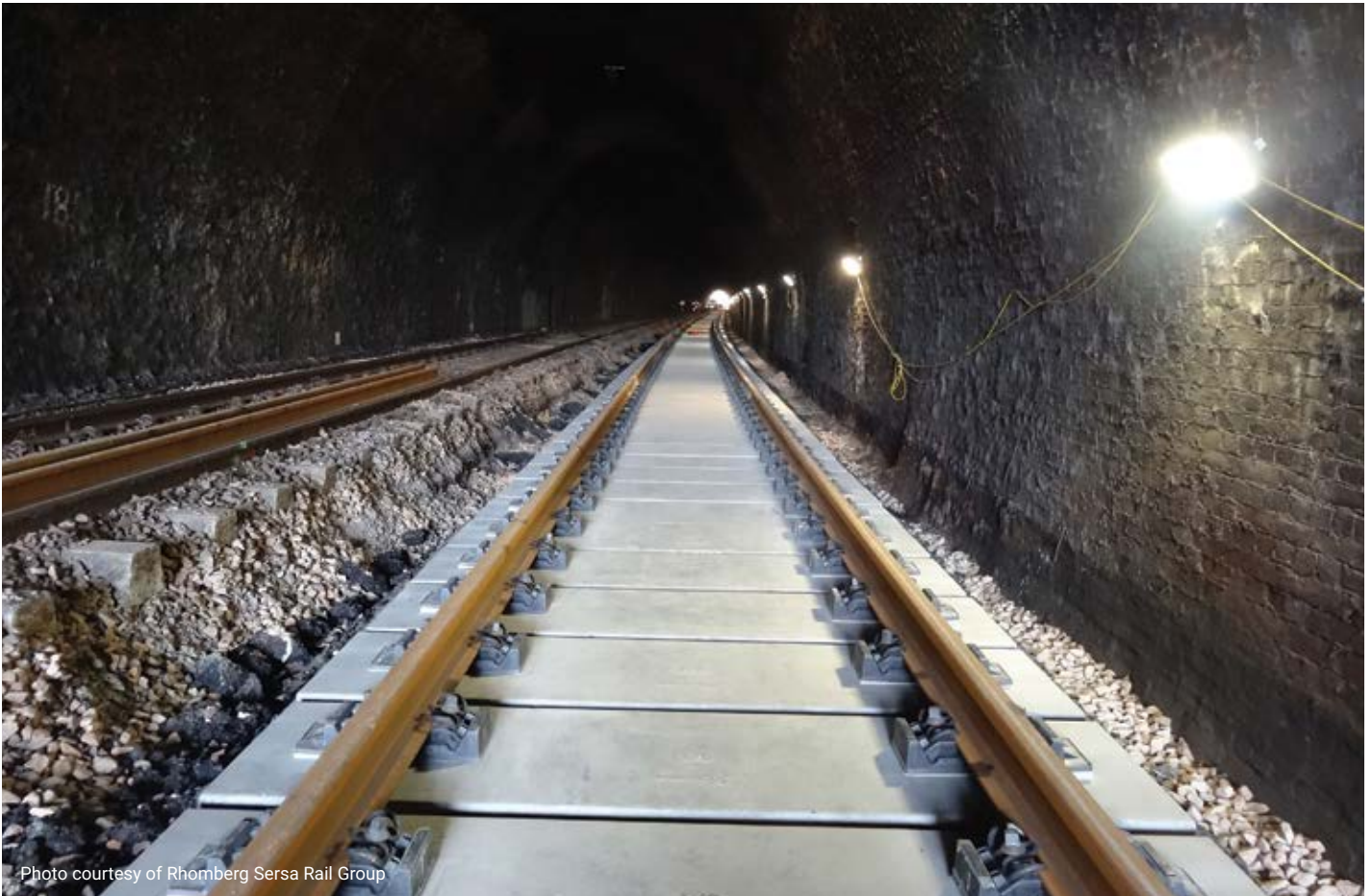
Workers installed approximately 800 feet of IVES precast slab track at Asfordby Tunnel in the U.K.
