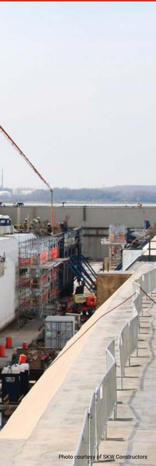
Workers pour concrete for one of the tunnel's 11 massive precast segments.
