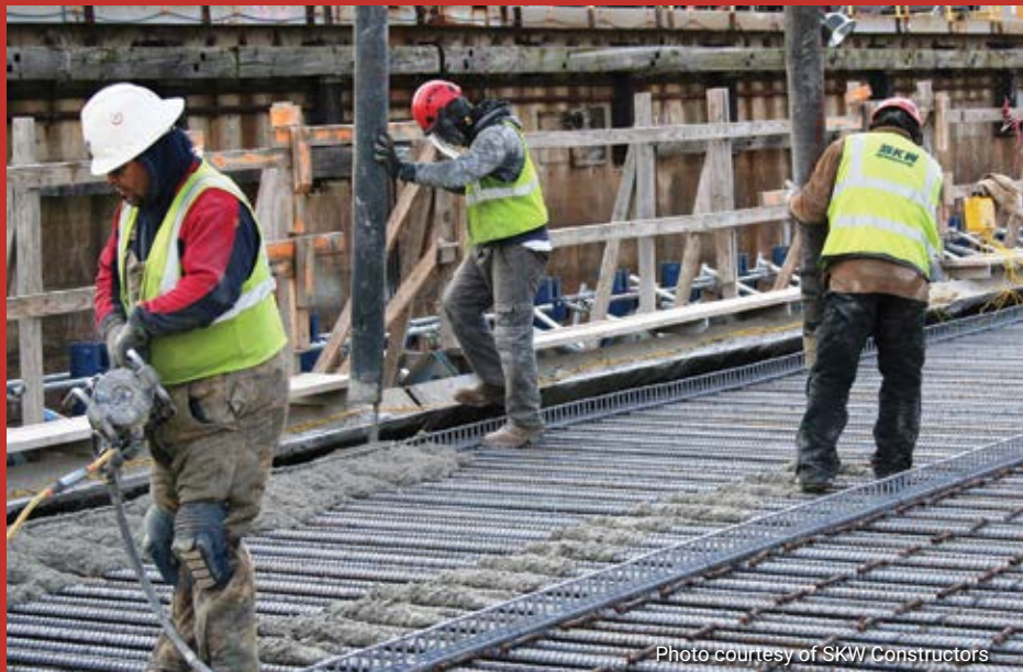
Workers pour concrete for one of the tunnel's 11 massive precast segments.
