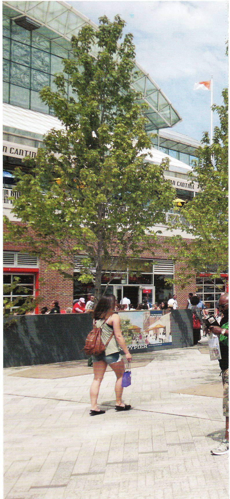
The installation of 59 massive precast concrete tree pits helps enhance the visitor experience at Chicago's Navy Pier.
