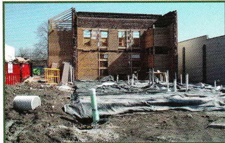
During construction of 347 S. 8th Street
